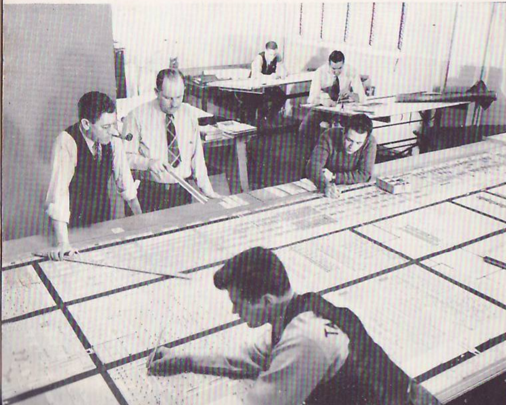
The tank which whipped Rommel, the M-3. Note the two cannon, the larger in a sponson on the lower right hand side. (Below) How Plant Engineering plans a factory. Every machine tool of the arsenal layout was spotted in this factory.
